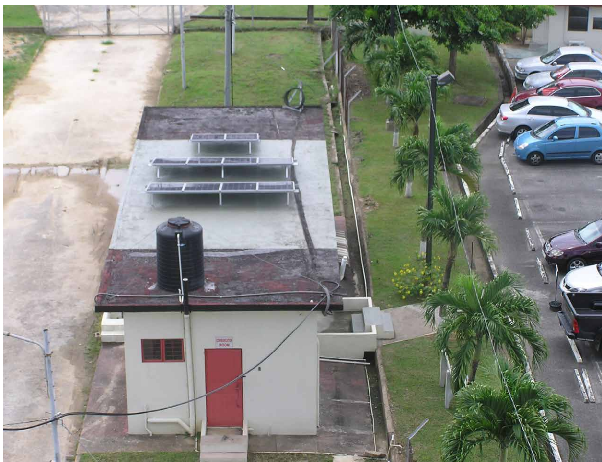
▲ Implementation of Grid tied Solar installation at T&TEC, Mt Hope, Trinidad. 10 PV panels were installed, 2012
